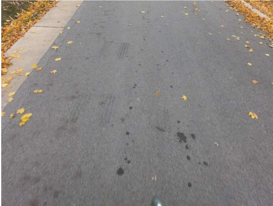
PASER 7 – Hudson Avenue (Richmond Ave to Western Ave)
